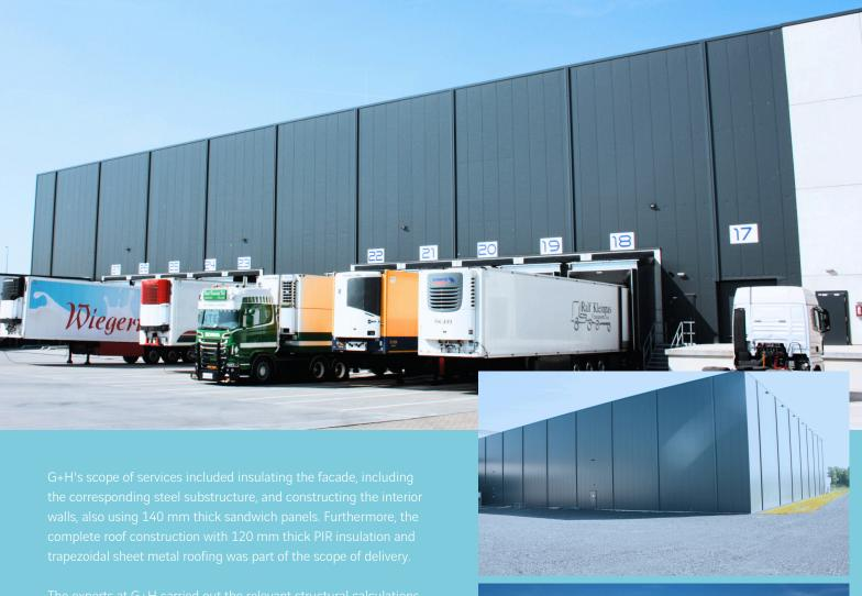
The experts at G+H carried out the relevant structural calculations for the facade and roof covering. To ensure that the construction project remained on schedule, up to 18 fitters worked on the new building every day.
