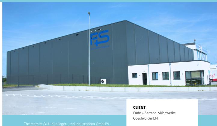
The team at G+H Kühllager- und Industriebau GmbH's Münster branch has expanded storage capacity at the Coesfeld site for Fude + Serrahn Milchwerke GmbH. Work on the warehouse took eight months. A three-part warehouse was created, consisting of a cold store, packaging materials warehouse, and transport corridor. In addition to expanding storage capacity for finished products and packaging materials, the packaging warehouse is now also equipped for later use as a cold storage facility.
