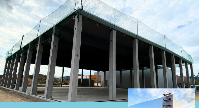
Petfood opted for precast reinforced concrete elements as the supporting structure for the new deep-freeze warehouse. All compo-nents, such as HTU and HTA rails for fastening the exterior panels and the roof structure, were installed in accordance with G+H's structural specifications. The gable roof was constructed from trapezoidal sheets with appropriate insulation and waterproofing.
